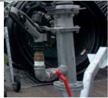
Second sprinkler on the trolley
